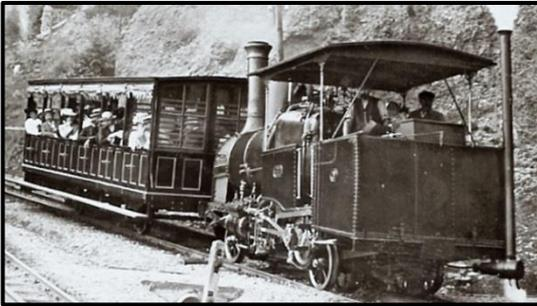
**Figure 6: Rigi rack-and-pinion railway**
